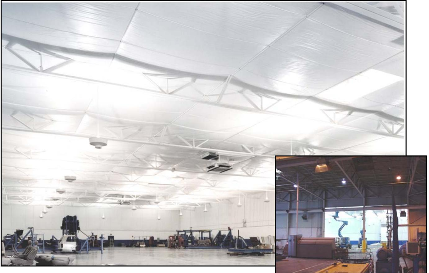
Commercial Building & Retrofit, Inc. is a sister company to BEST Lights. We took this 42,000 sq. ft. building and turned it into a energy efficient testing facility for MGA Research. We started with insulating the ceiling and walls to a R-19 then lit the facility with glare free 1000 watt MH-IBU indirect BEST Lights.
